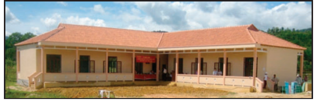
Team XXIII—Completed A Dot primary school
