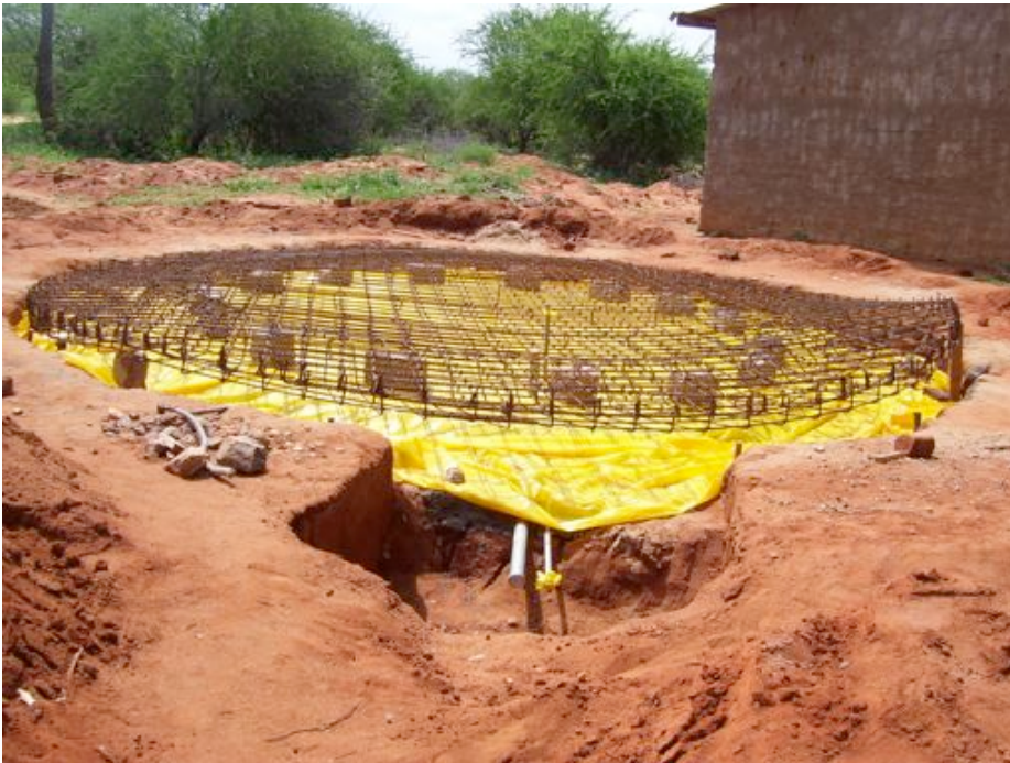
Foundation for the 1 st collection tank in progress
