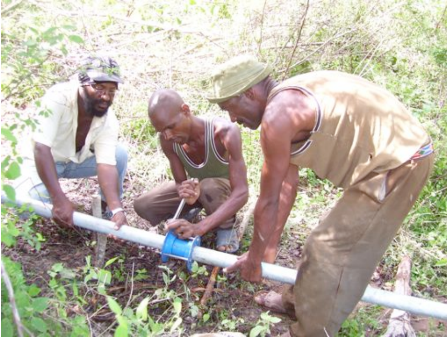
Plumbers connecting the GI pipes
