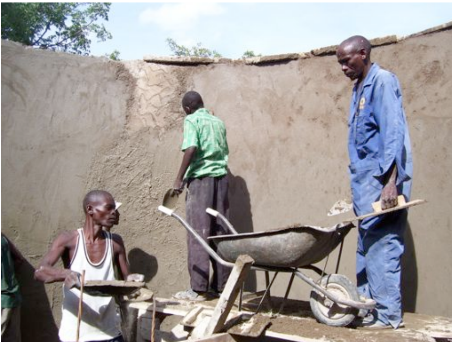
Masons plastering the inside of the 1 st collection tank
