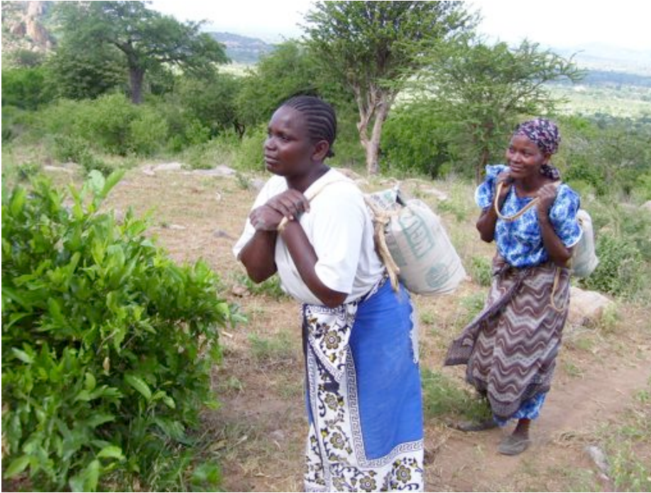
Women ferrying cement in preparation for the 2 nd tank – 25m 3
