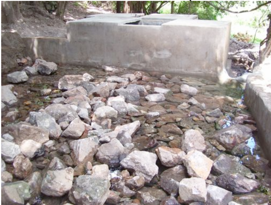
Completed Intake Chambers & Weir
