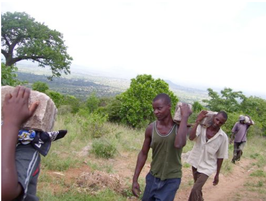
Some community members ferrying materials uphill for the 1 st collection tank
